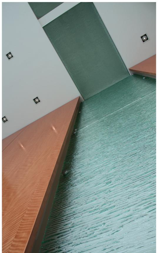
Texture: MD230 Neo Strata 1/2" Clear Tempered Kiln-Fired Glass 1/2" Clear Laminated Kiln-Fired Glass
