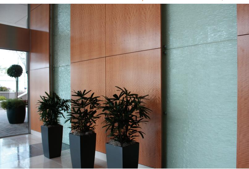
Texture: MD230 Neo Strata 1/2" Clear Tempered Kiln-Fired Glass 1/2" Clear Laminated Kiln-Fired Glass
