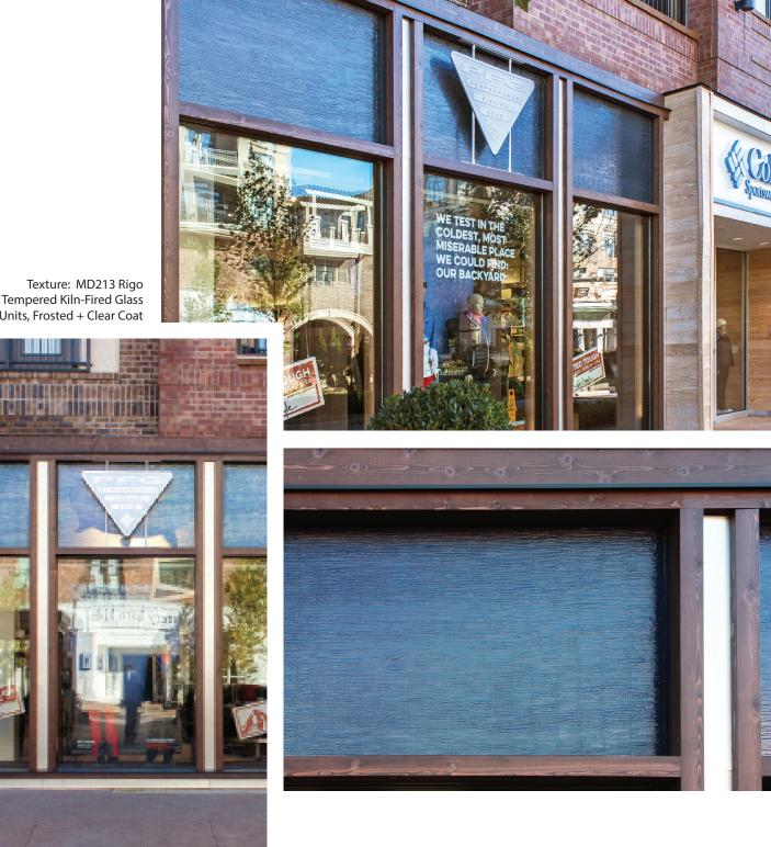
1" Tinted Solar Blue Tempered Kiln-Fired Glass Insulated Units, Frosted + Clear Coat
