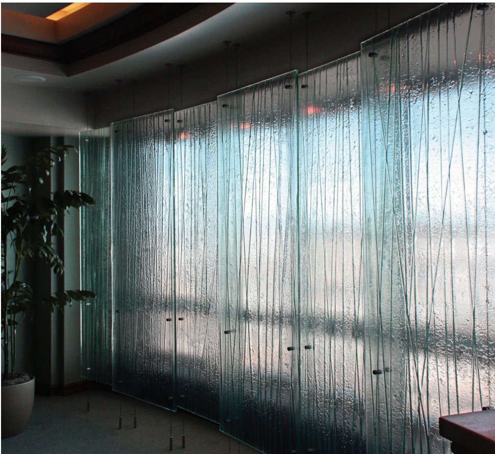
Texture: Custom Texture 1/2" Clear Tempered Kiln-Fired Glass
