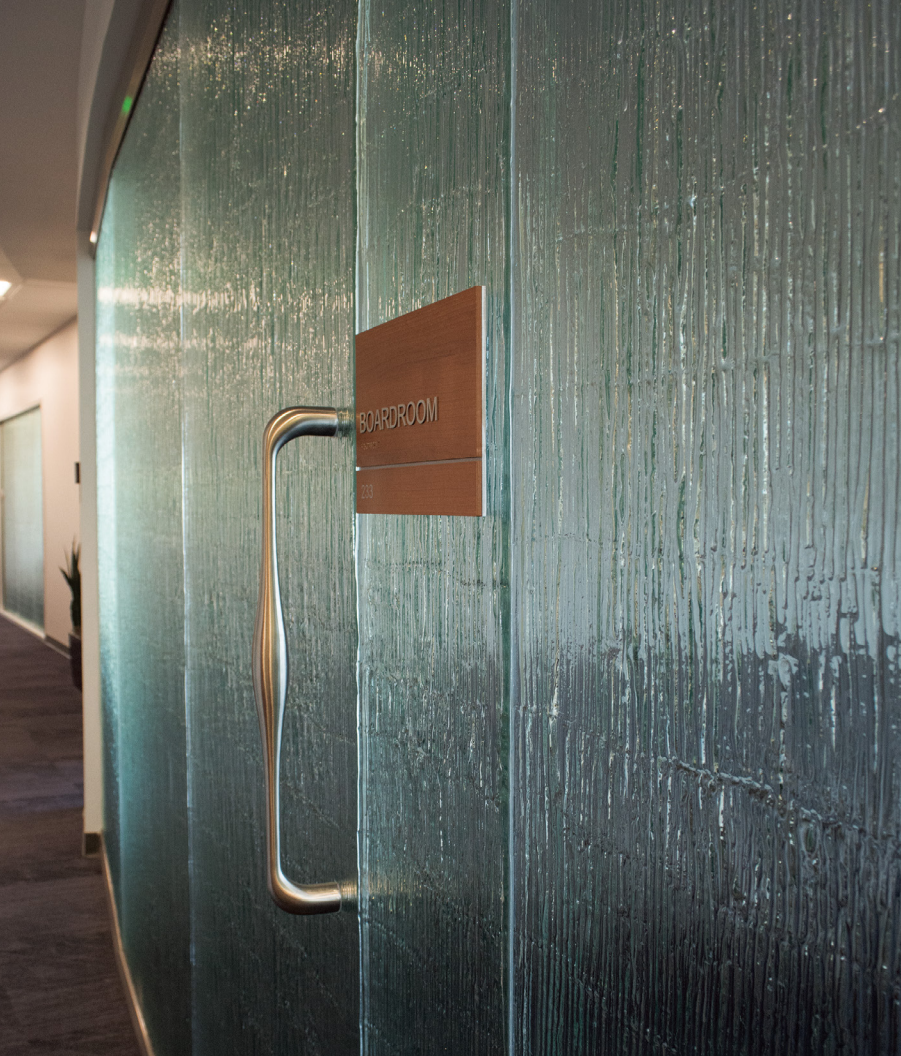
Texture: MD213 Rigo 1/2" Clear Tempered Kiln-Fired Glass
