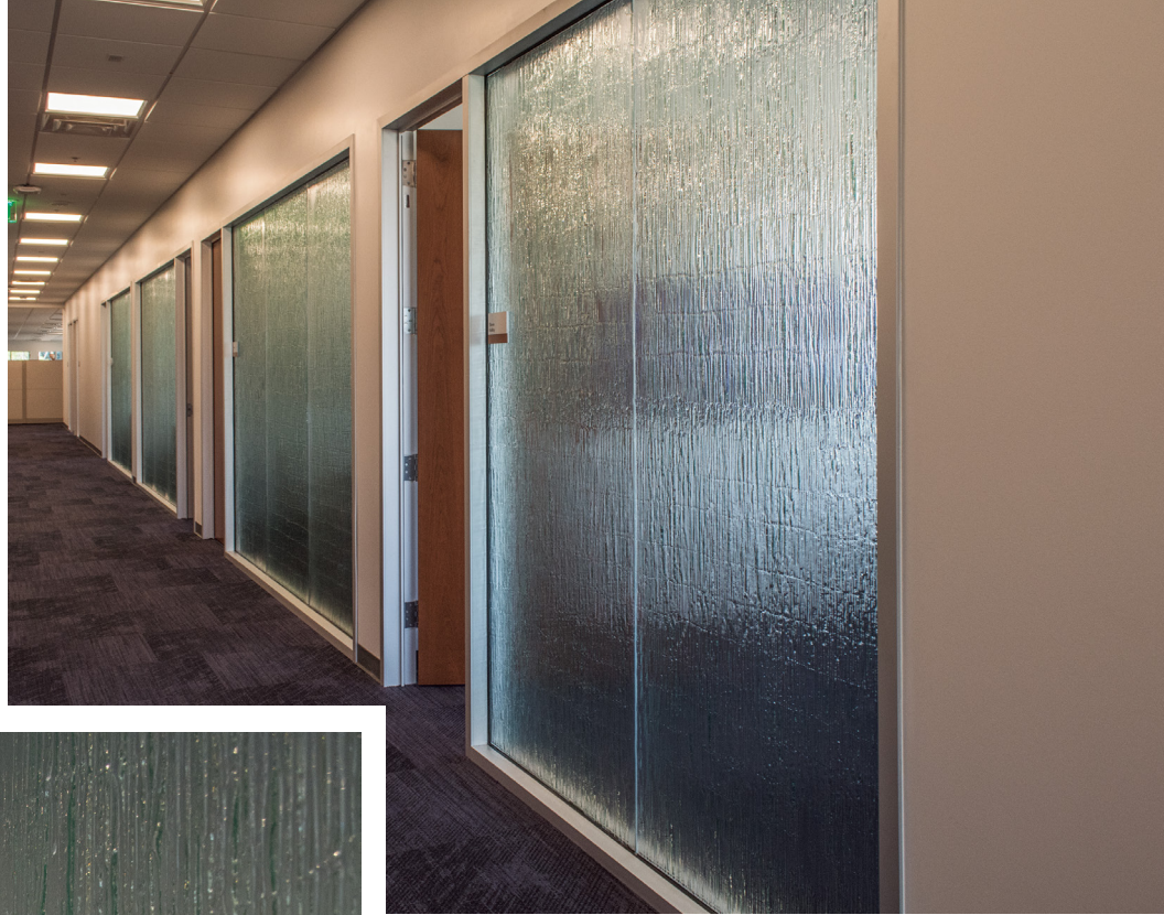
Texture: MD213 Rigo 1/2" Clear Tempered Kiln-Fired Glass
