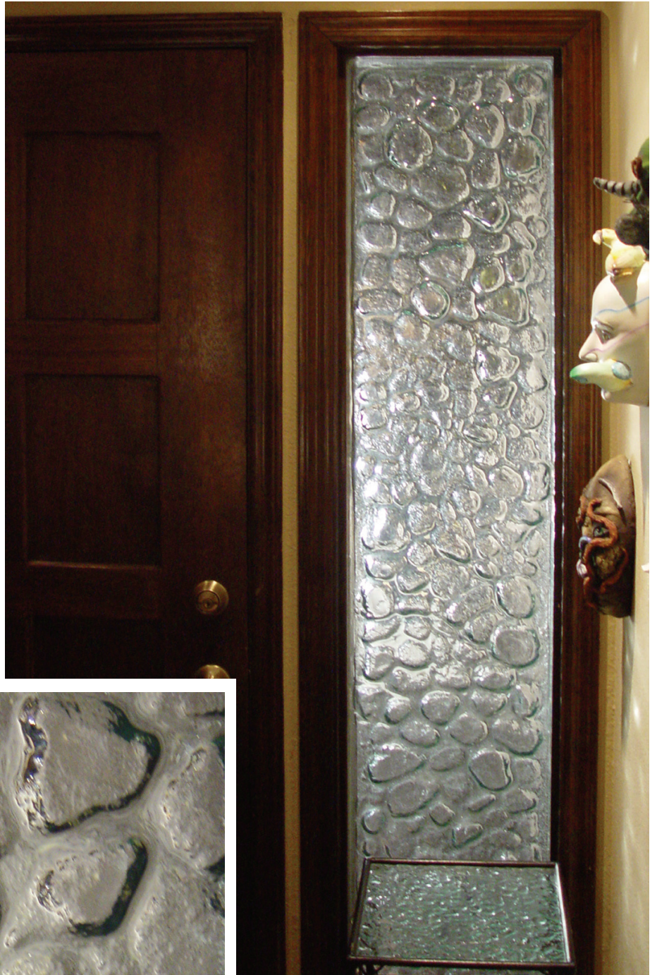
Texture: Custom Texture 1/2" Starphire Tempered Kiln-Fired Glass
